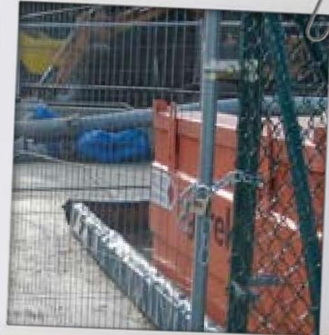
Secured fuel tank in secondary containment
